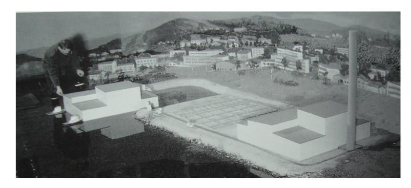
4x190 MW plant was designed in 1989 for Norway by IVO Size of largest module: 40 m long, 58 m wide, 8000 tons No permission was given because of CO2-emissions
